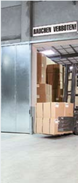
6 Fire sliding doors
