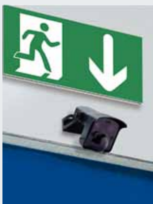
Radar detector in escape direction as standard
